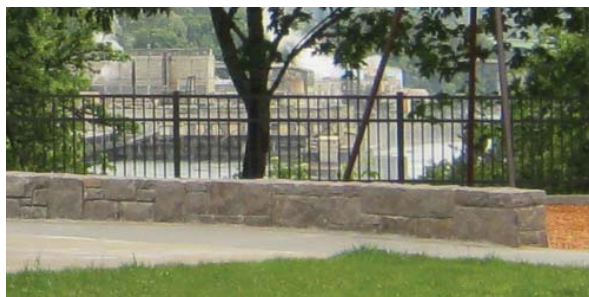
Low Retaining / Seat Wall
