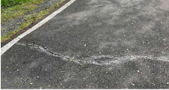
Trail surface uplift from tree roots
