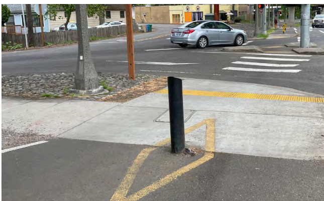
Bollard without reflectors
