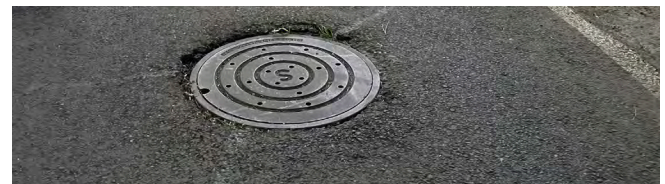
Uneven manhole cover
